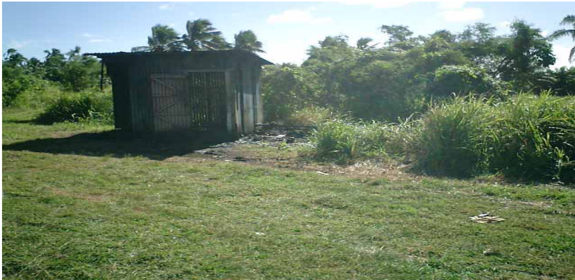
Photo: 3 Showing pump sheds in Nuku'alofa Bore well field.(Davendra Nath- SOPAC)
