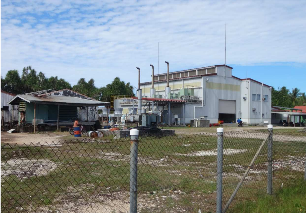
Figure 2: Fogafale Power Station
