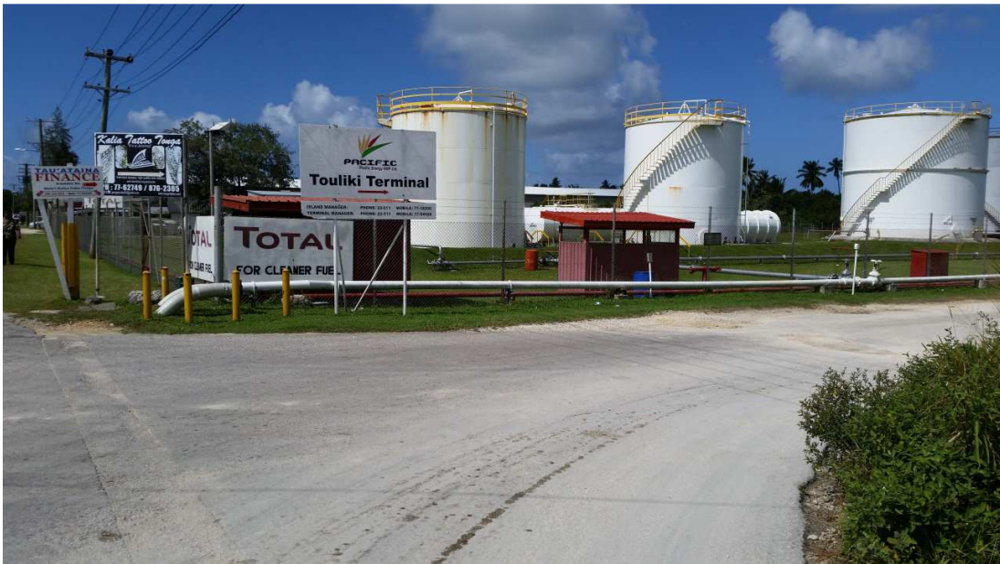
Figure 2: Oil Companies Terminal
