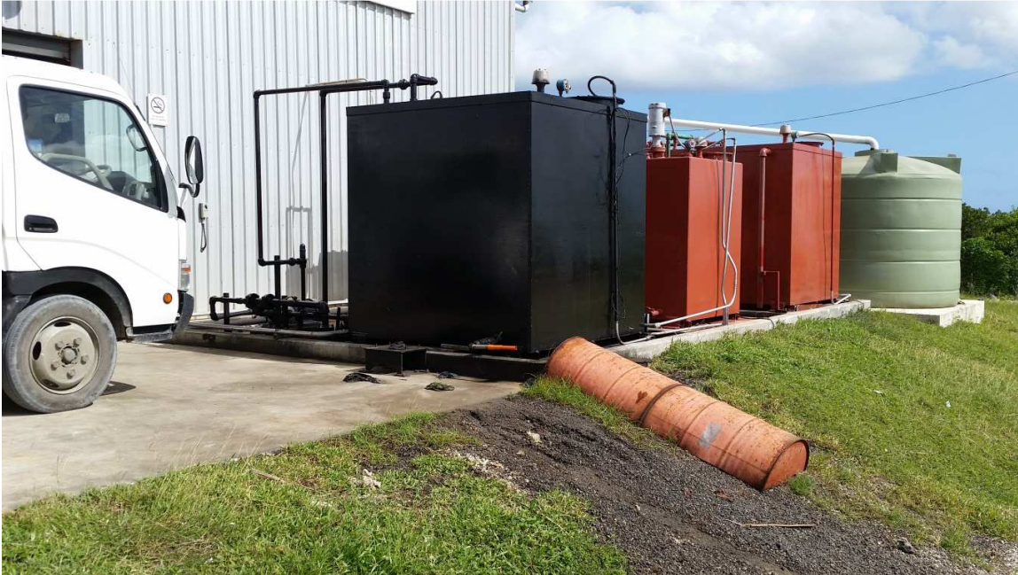
Figure 4: Point of Waste Oil Fillings– TPL Popua Power Station
