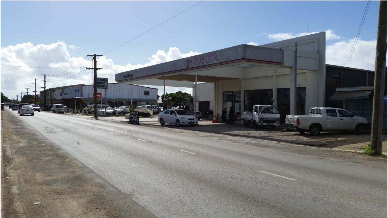
Figure 6: Asco Motors station service
