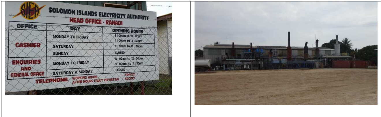
Figure 2: SIEA and the main Power station at Lungga Power Station (near the Airport)
