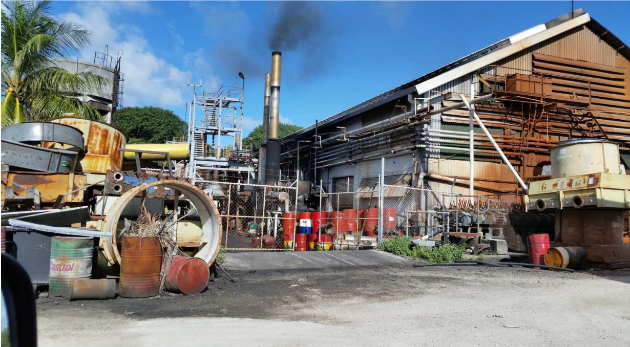
Figure 5: Current storage on site (power house)
