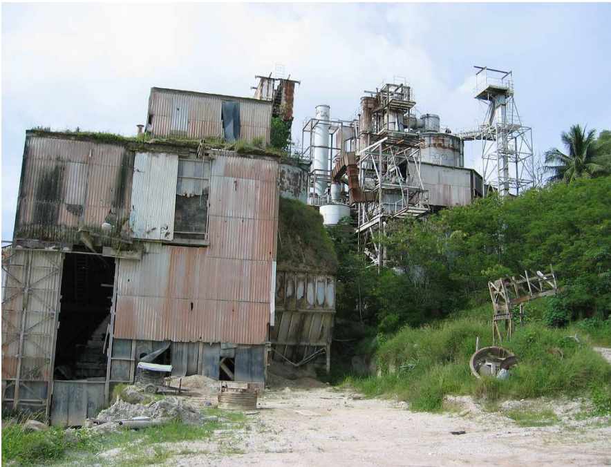
Figure 3: Old phosphates treatment plant
