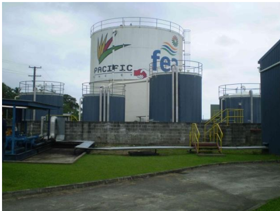
Photo 1 - Kinoya Tank Farm
