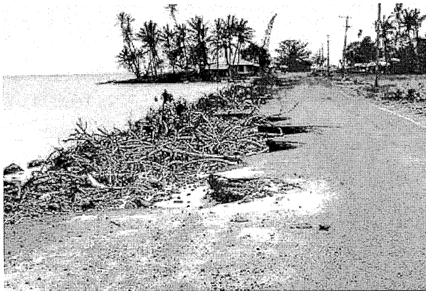
Figure 1. Coastal erosion affecting infrastructure, including the house in the background (photograph from Beca International)
