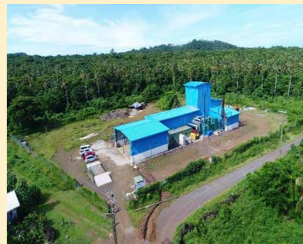
Afolau 750kW Biomass Gasification Plant on STEC lands at Mulifanua.
