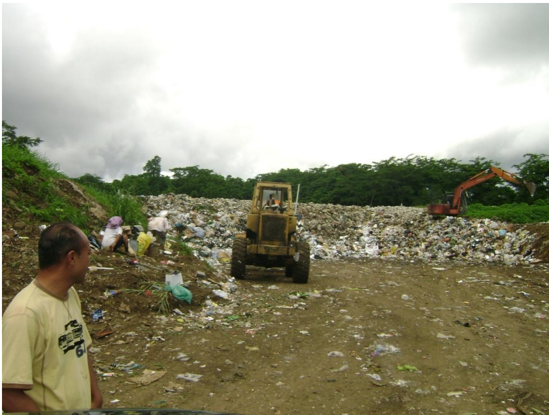
Figure 7: One of the waste cells at Tafaigata Landfill
