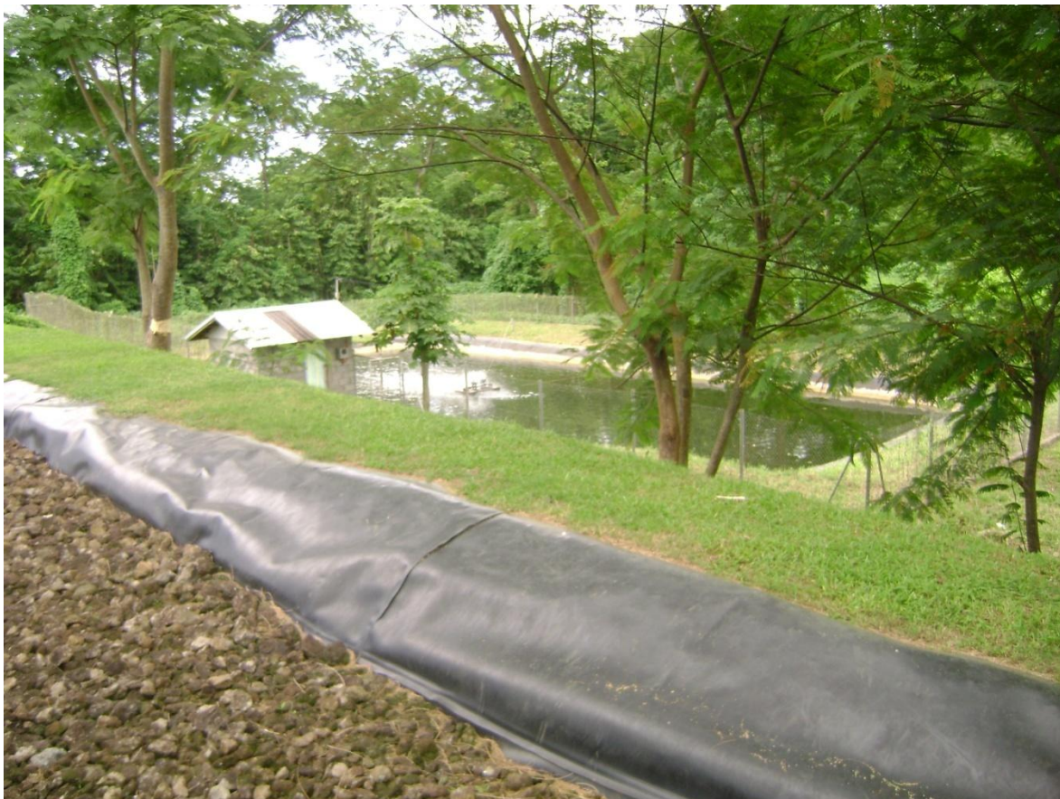
Figure 8: Leachate facility at Tafaigata landfill
