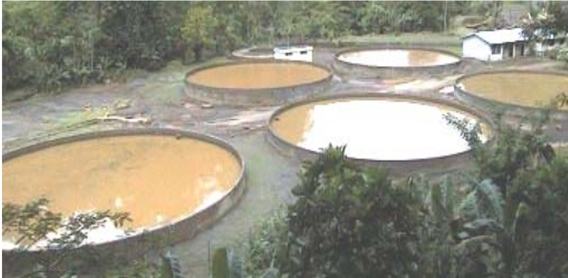
Figure 3.5: Impact of flooding on water reserve tanks
