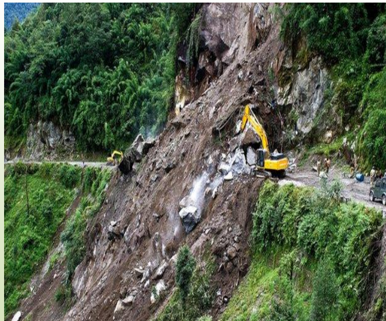
Figure 13: Example of the impact of a land degradation activity - landslide on a road without stabilization of the steep slopes it is located. Source: MNRE
