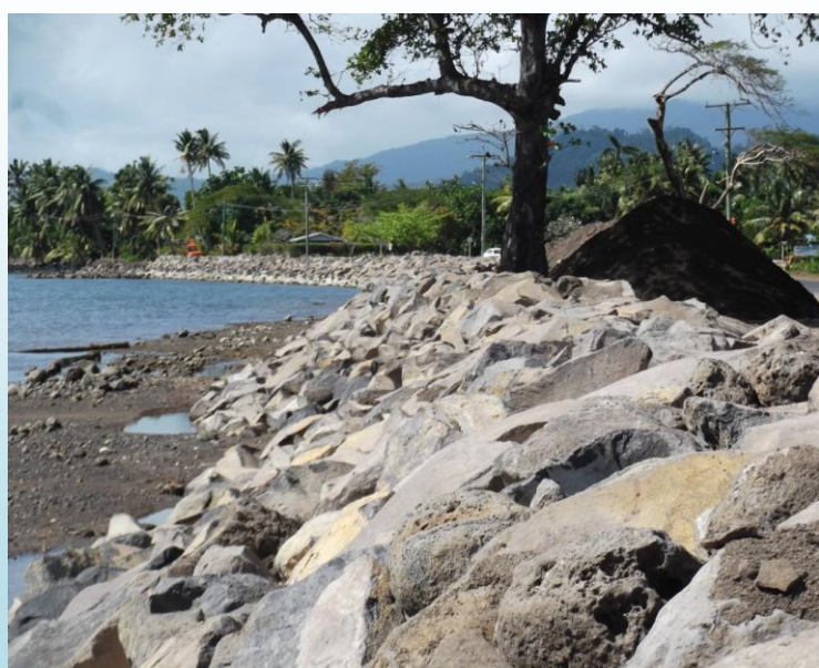
Figure 16: Example of an extensive seawall project - Vaiala Upolu Island. Source: MNRE.
