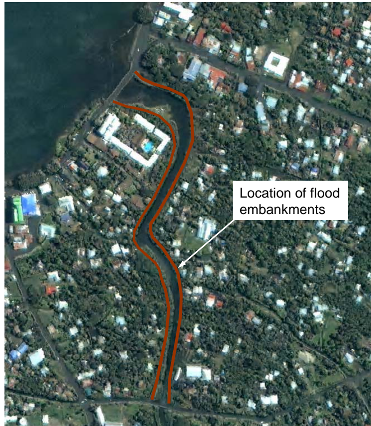
Figure 3-2: Location of flood embankments for the lower Vaisigano River downstream of Leone Bridge
