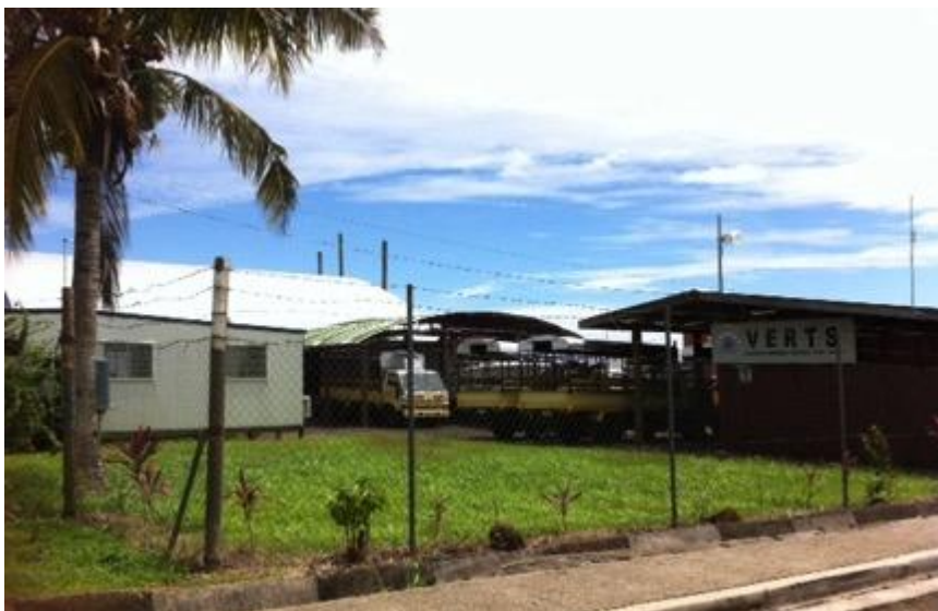
Figure 13 Existing block of land for NEOC office in Samoa
