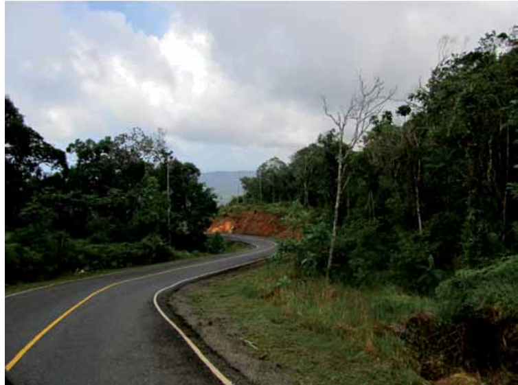
Development projects such as this road through Gunayala protected area (managed by the Guna people), Panama, should be subjected to free prior informed consent © Onel Masardule
