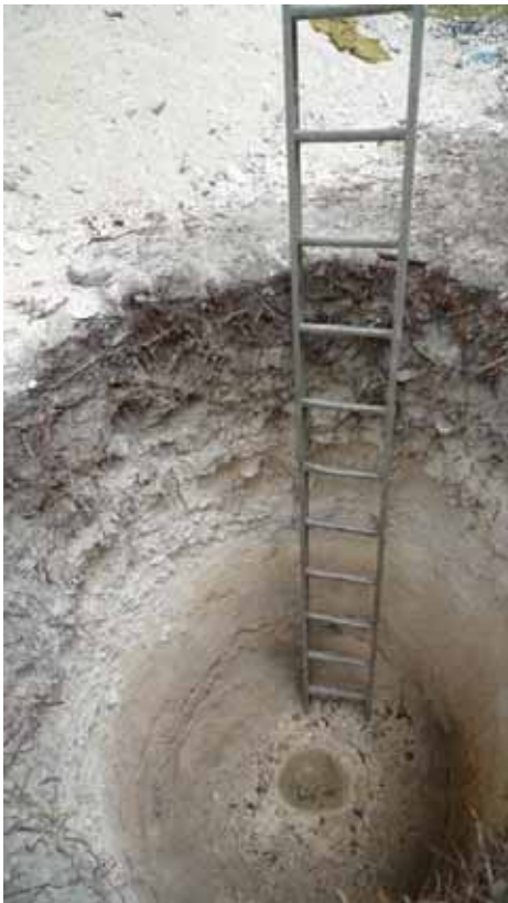
Plate 32. Well under construction in response to shortage of water - Vaitupu
