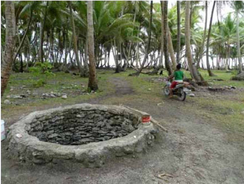
Plate 27. Traditional well - Vaitupu used for washing and watering pigs (note corn beef tin on pole as means of abstracting water).
