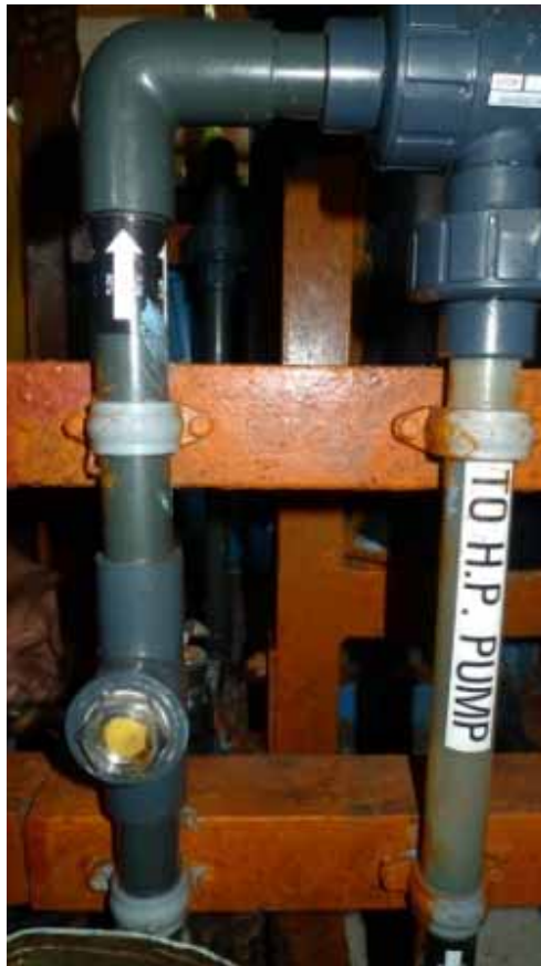
Plate 18 Fittings for installing pressure gauges for product water and brine water
