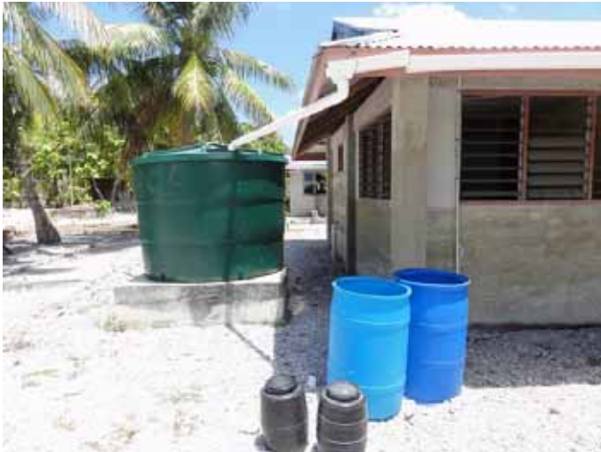
Plate 39. Rainwater harvesting - Niutao. Note the 200L containers to collect the water from an inefficient gutter.
