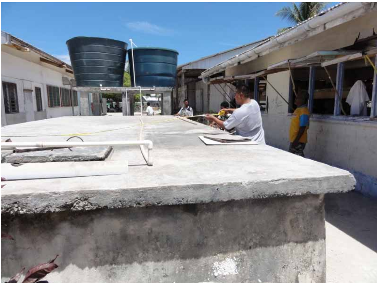
Plate 28. Measuring Rainwater Cistern - Motufoua High School - Vaitupu Island
