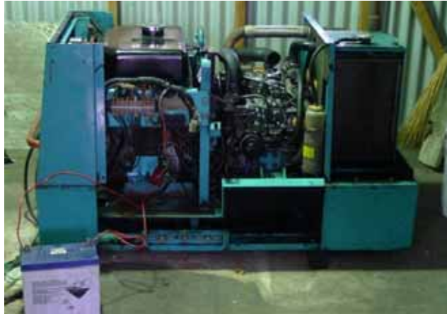
Plate 11 Generator used for desalination plant - requires new cooling system
