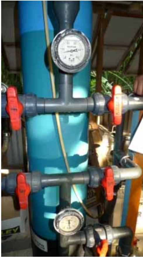
Plate 15 Pressure meters for sand filter required
