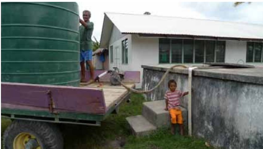
Plate 26. Pumping from communal cistern for water distribution - Vaitupu
