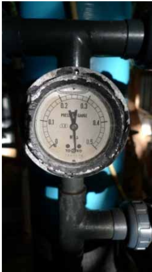
Plate 14 Pressure meter for sand filter required
