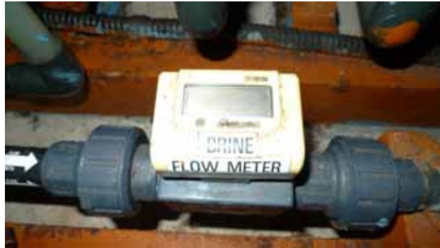
Plate 13 Flow meter for brine and product water required
