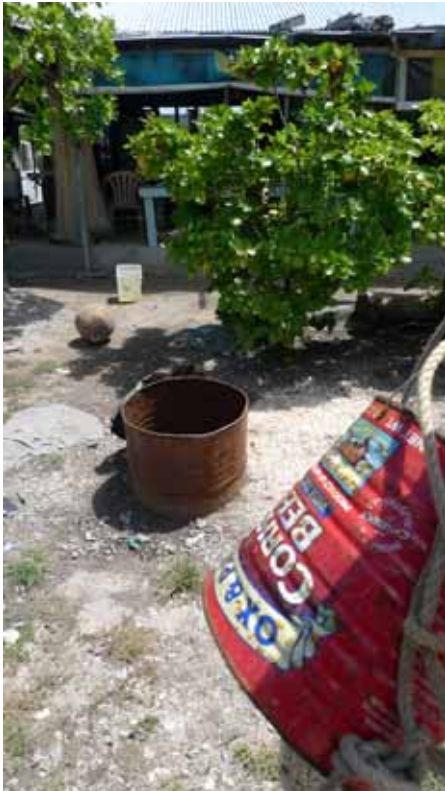
Plate 31. Domestic well, 44 gallon drums for casing, with corned beef tin used as a bucket for extracting water - Nanumea
