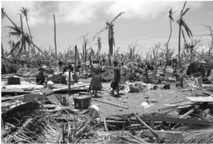
Figure 7. Houses were blown apart by Typhoon Maysak, their contents strewn in the wreckage of trees on Ulithi atoll. (Photograph supplied to Australian Broadcasting Corporation by Brad Holland, freelance photographer and Co-chair of the American Society of Illustrators Partnership.)
