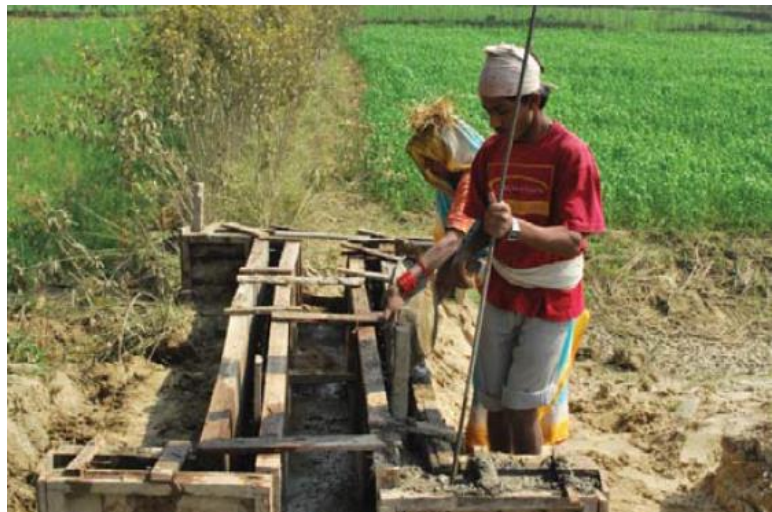
Construction and maintenance of irrigation canals (ILO, 2011)
