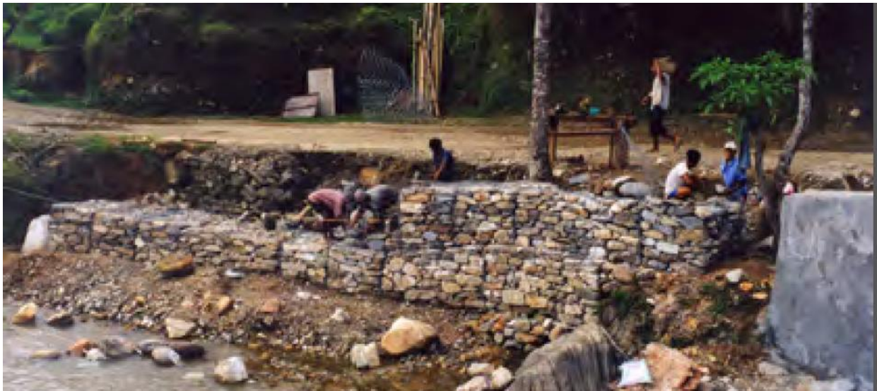
Flood control works (ILO, 2011)
