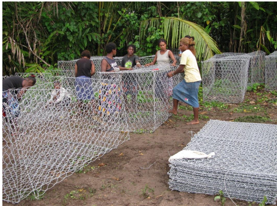
Women in the Solomon Islands (Malaita Province) making gabion baskets for the SIRIP Project (ADB, 2010)
