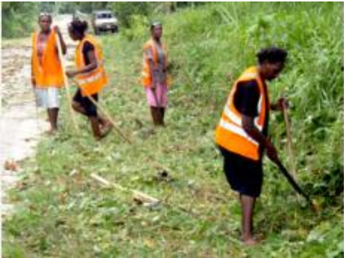
Photos: Road maintenance (ADB, SIRIP)
