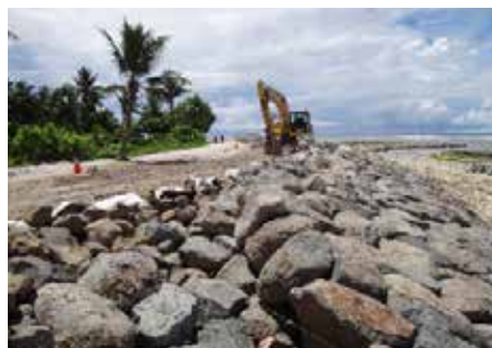
Photo 2: Rock revetments (Shand) in Kiribati
