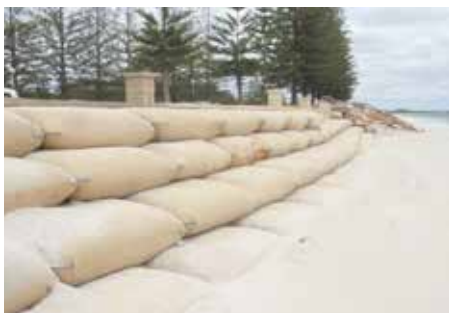
Photo 1: Semi-rigid geotextile container (Maccaferri NZ Ltd.)
