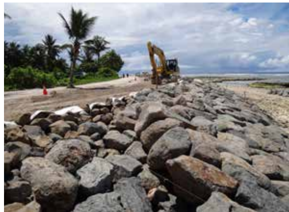
Photo 12: Rock revetment
