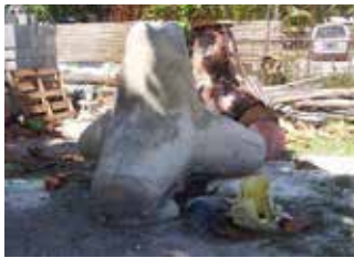
2T Tetrapod unit cast in Kiribati (source: I-Kiribati, 2013)
