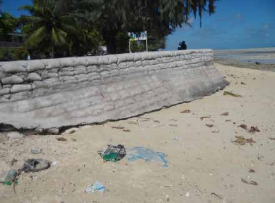
Photo 7: Grout-filled sandbags (Credit: Shand 2015)
