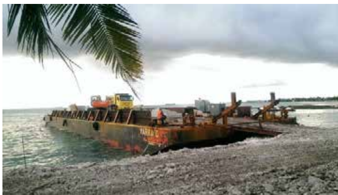
Photo 21: Example of barge unloading gravel for replenishment at Tuvalu. (Source: taiwanembassy.org)
