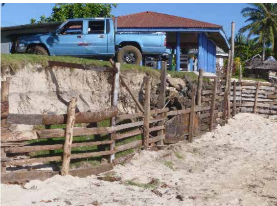
Photo 13: Rock filled timber wall
