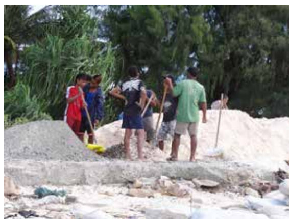
Photo 19 and Photo 20: Local coral aggregates being supplied and mixed by hand in Kiribati, 2015 (Credit: Shand)
