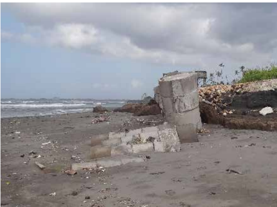
Photo 11: Concrete filled drums
