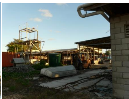
Photo: Metal building 'skeleton' in shipyard.
