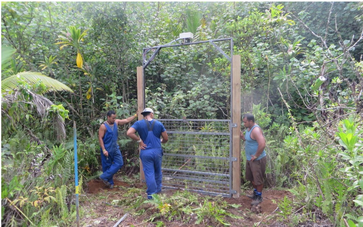
Construction of the lured enclosure drop-gate, showing electronic gate trigger at top
