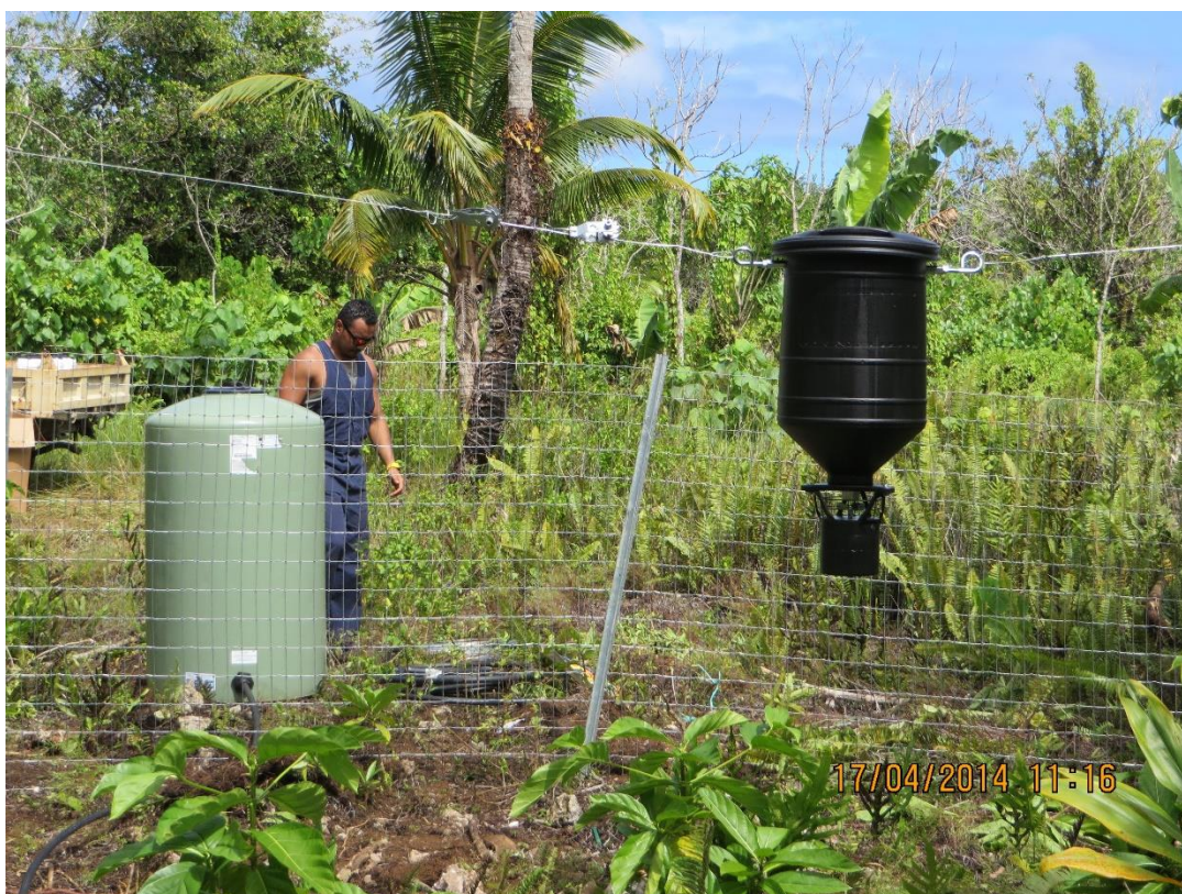
Construction of lured enclosure, showing automatic feeder and water tank to supply trough
