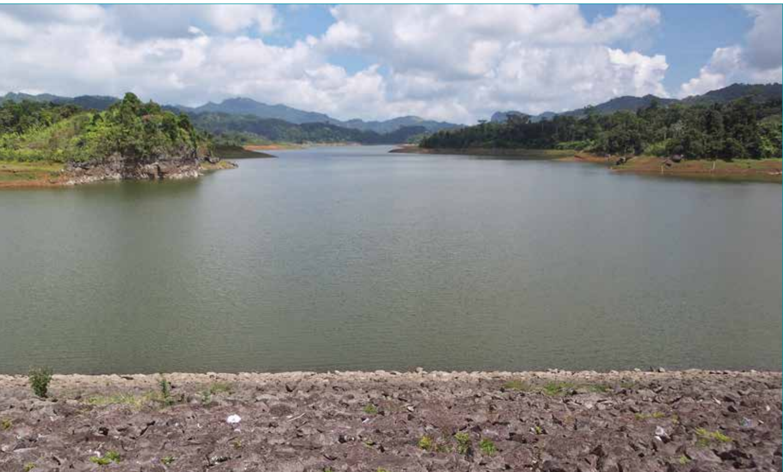
Monasavu Dam. Photo: Adil Ali, Fiji Meteorological Service
