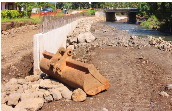
Construction of a revetment wall Vaisigano River
