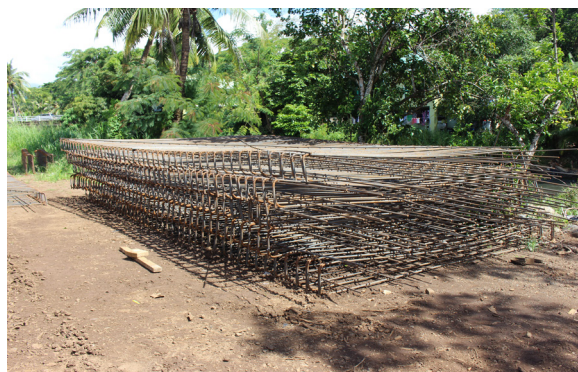
Rebar beams for the river wall foundation
