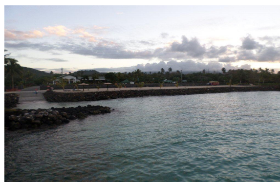
Reclamation at Suifaga - Amoa Resort
