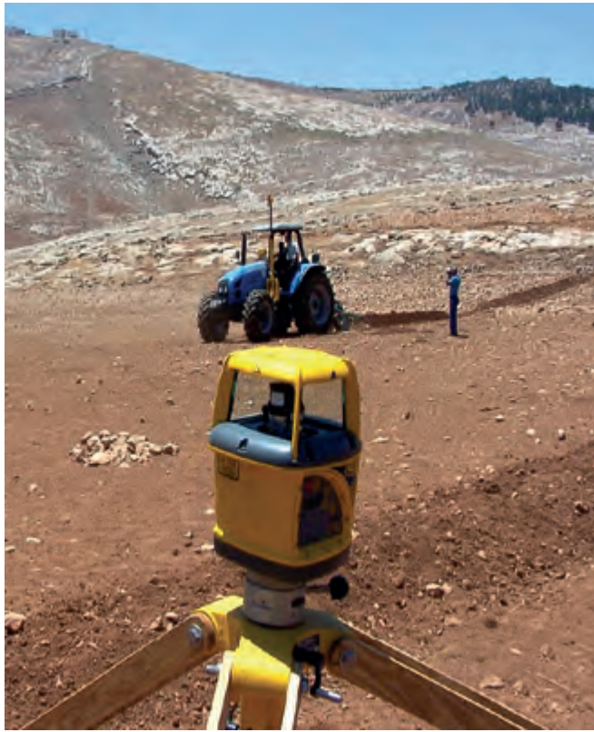
Greening the Badia: laser-guiding micro-catchment water harvesting technology on contours for forage shrubs
