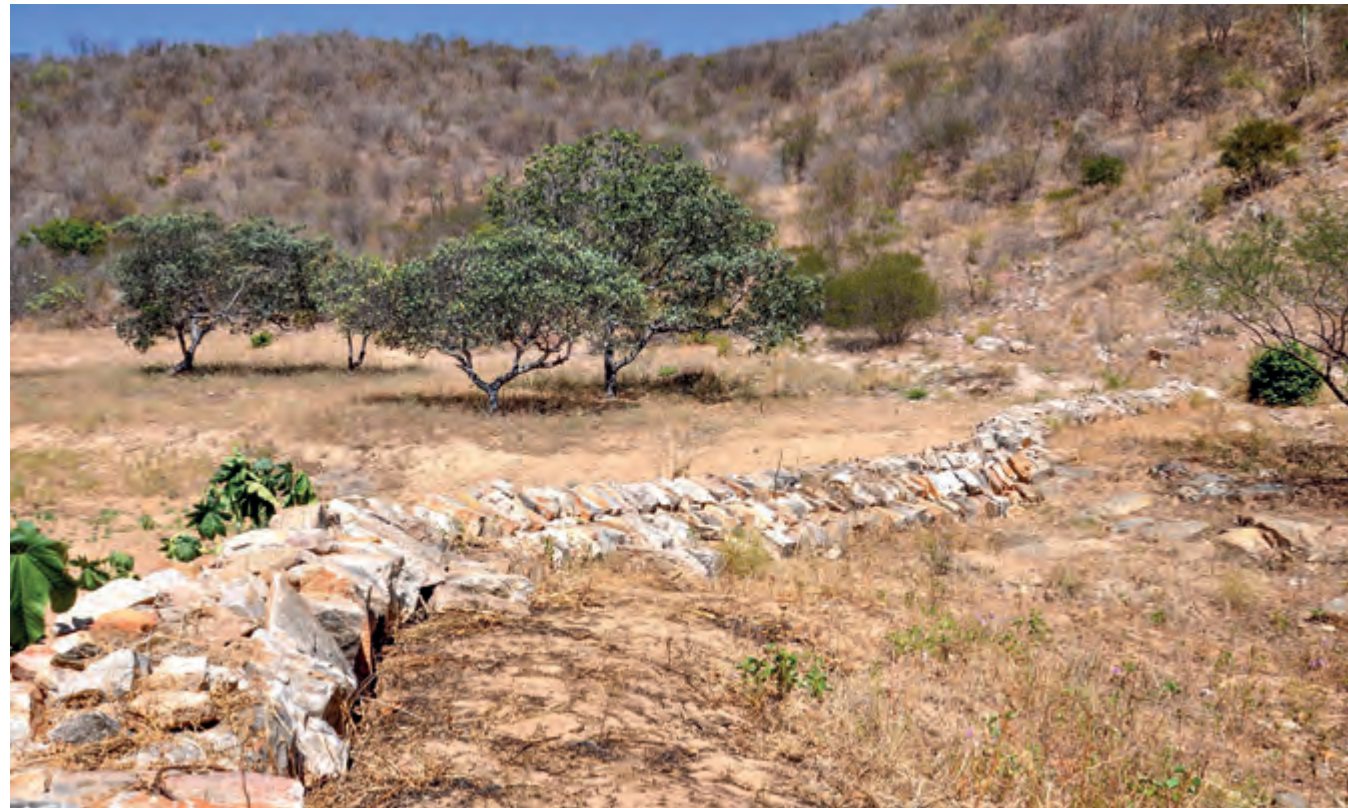
Successive sediment containment barriers, ensuring water retention in the soil and a productive environment
