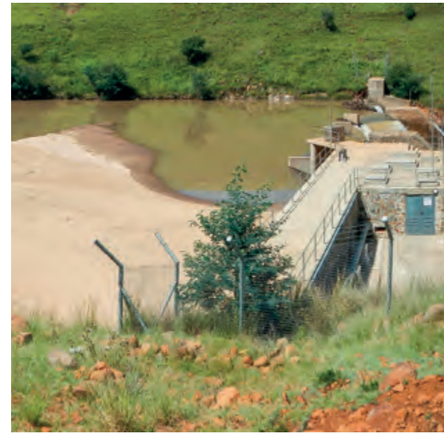
The silted-up dam at Mount Fletcher
