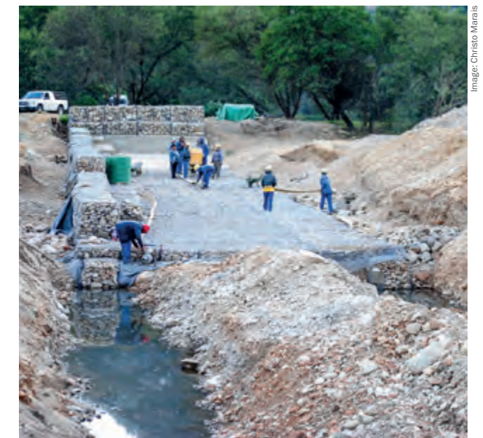
Workers restoring a highly degraded wetland in the Baviaanskloof
