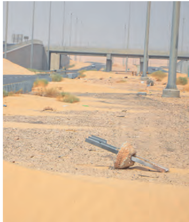
Two field photos showing severe sand encroachment along Sabiyah Road
