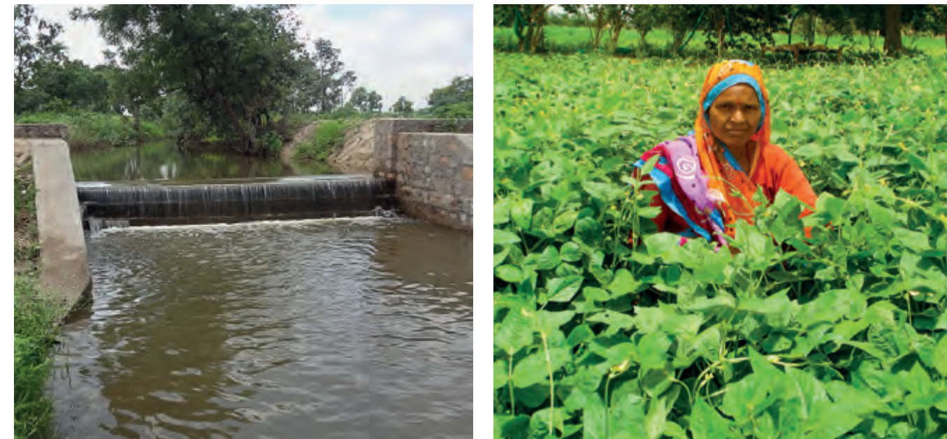
Parasai-Sindh watershed, Bundelkhand region, central India: (left) over and base flow from a check-dam indicates increased groundwater and surface water availability; (right) farmer cultivating vegetable as cash crop
