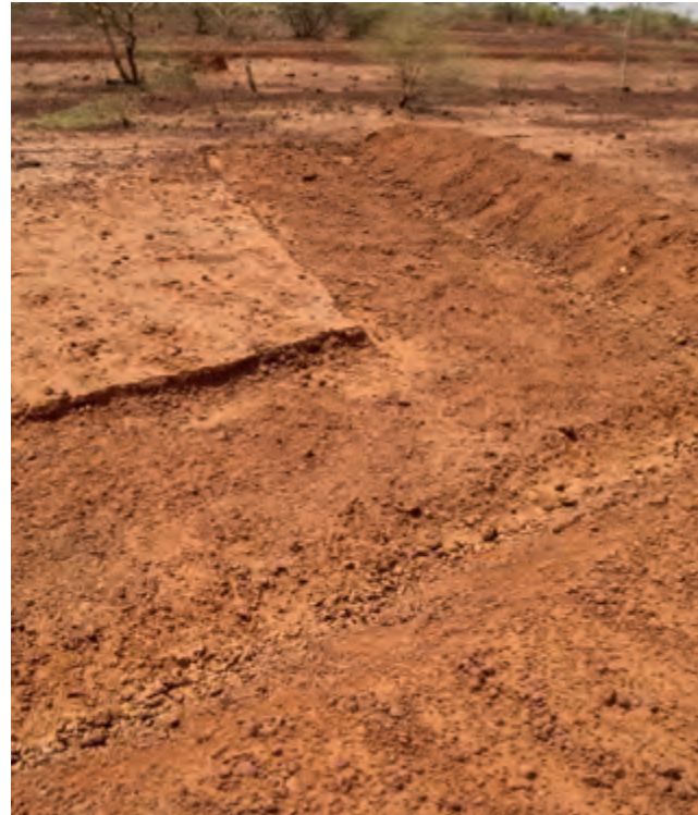
Glaze treatment methods include benches to control erosion, like these ones at Yettoré Allah, Niger
