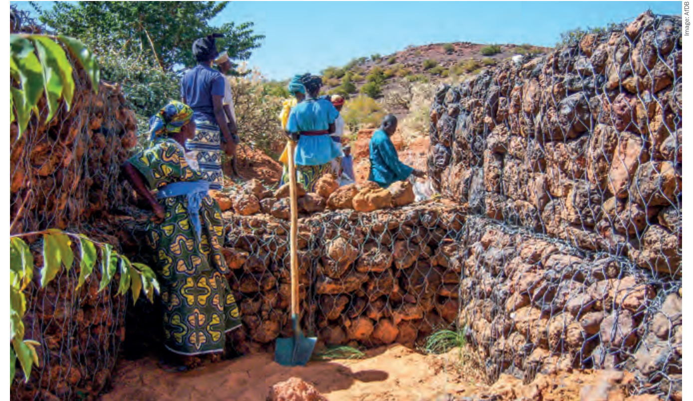
Thresholds of gabion and dry stone in the Tillabery region, Niger
