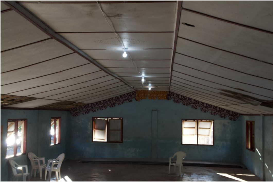
The following day, the remaining three buildings were electrified the same way and also tested.
