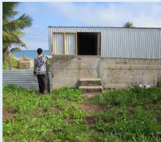
Kuilani Fa'asolo of Caritas Tonga inspects a newly completed water tank in Ha'apai, in August 2016.
