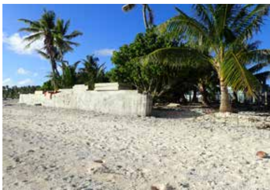
The end of the wall in progress.
