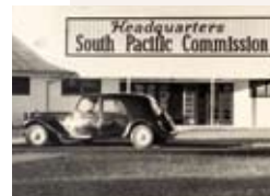
The Pentagon's headquarters in Noumea during World War Two became the head office of the Secretariat of the South Pacific Commission (SPC). Photo taken in 1951.
