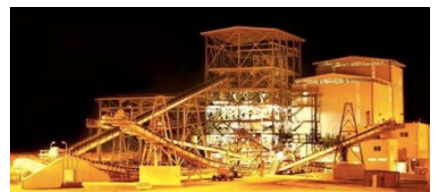
Mine infrastructure lit up at night, New Caledonia. Image © David Becker/SLN/ERAMET
