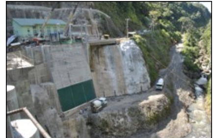
Construction of Nadarivatu dam in Fiji. Image © efl.com.fj
