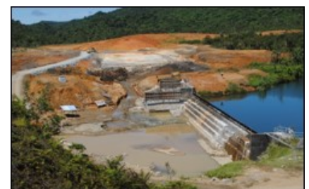
Construction of Wainisavulevu Weir Raising in Fiji. Image © efl.com.fj
