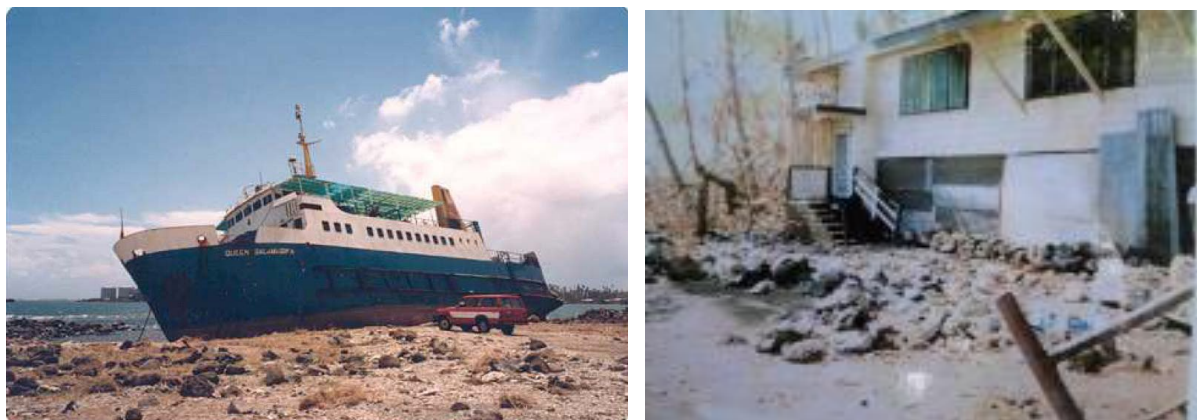
Figure 9. Damage in Apia caused by category 4 tropical cyclone Ofa : The beaching of the passenger/cargo ferry Queen Salamasina in Apia (left) and damage to houses (right).
