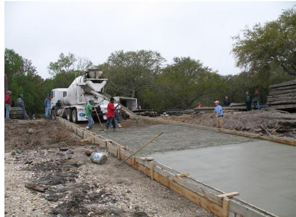
**Figure 9: Example of type of slipway being proposed and a deomstration of how the construction will proceed.**
