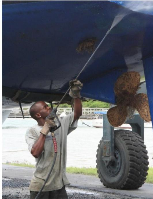
**Figure 11: Power washing of yacht hulls will be a frequent activity in the boatyard.**
