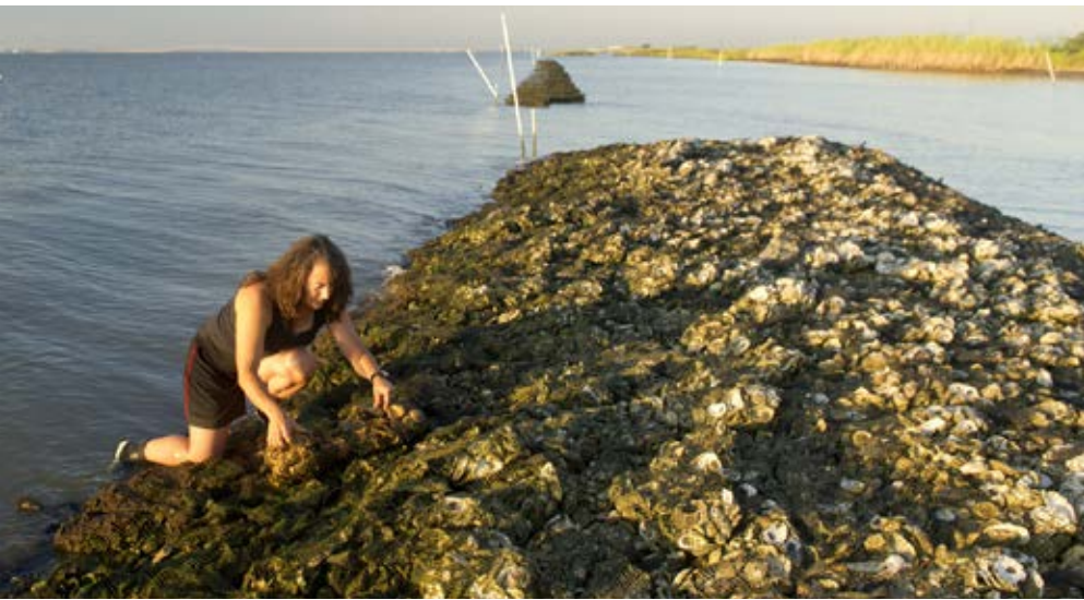
TNC scientist Judy Haner inspects a newly constructed oyster reef, designed to reduce coastal erosion, in Mobile Bay, Alabama, USA.
