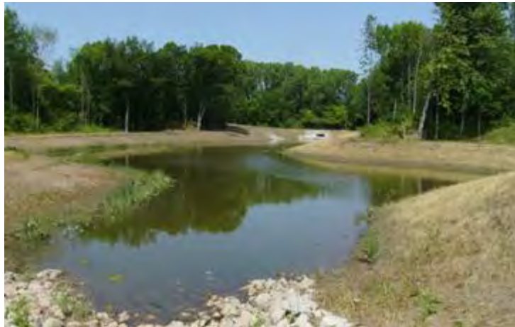
Figure 7.1. Typical man made retention pond
