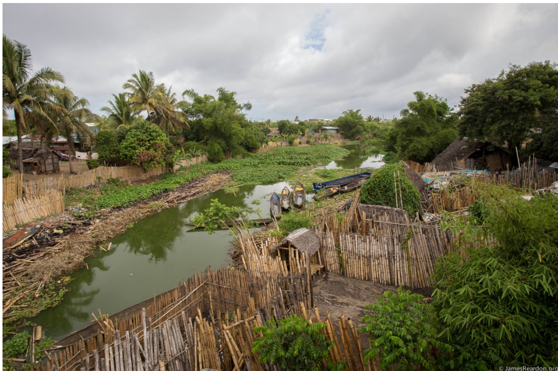
Fig. 3. Drainage channel in central Tamatave. Photo: J. Reardon.
