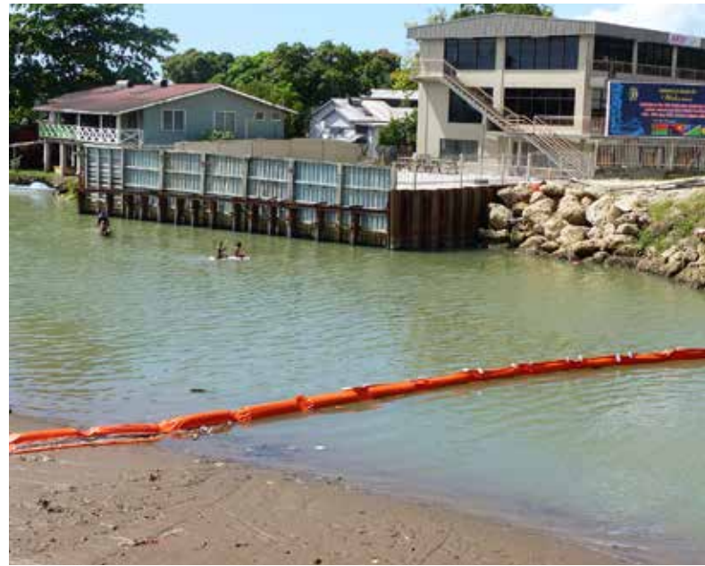
A river boom was laid across the Mataniko River in 2015 as part of the river clean-up project. Photo SPREP/L.Curry
