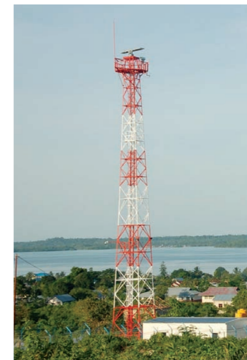
Figure 73: Surface radar for coastal surveillance (© Kelvin Hughes).
