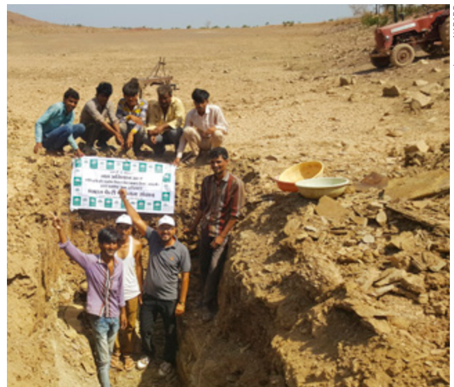
Digging a well, Gogharpura village, Mandasaur district, Madhya Pradesh
