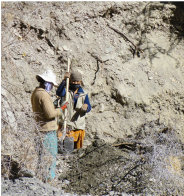
Digging an irrigation channel
