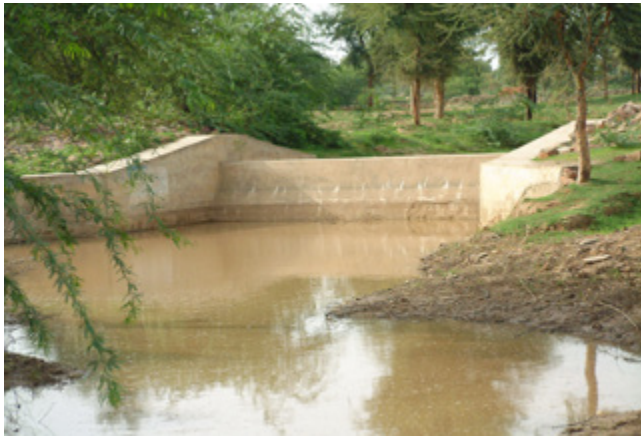
Various soil and water conservation structures at the Gokulpura-Goverdhanpura watershed. The soil and water conservation structures including 13 gabion structures (top left), 1,500 gully plugs, 34 loose boulder structures (top right), and 20 check dams (bottom left) were constructed in a watershed of 1,355 ha, which reduced the annual soil loss from 5.5 t/ha to 1.5 t/ha
