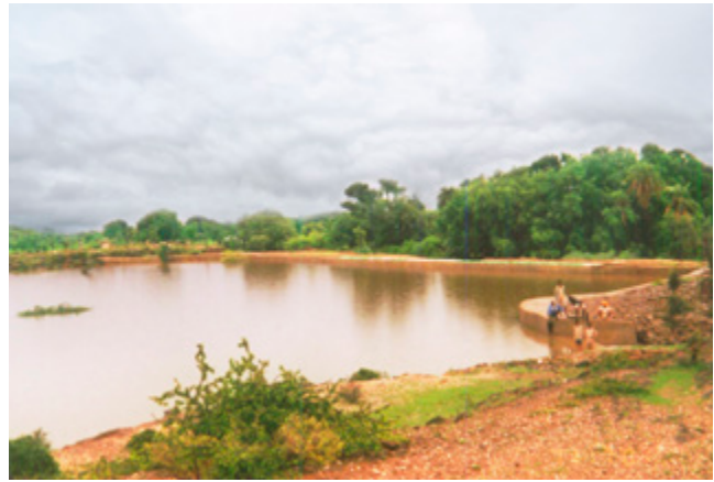
Various soil and water conservation structures at the Gokulpura-Goverdhanpura watershed. The soil and water conservation structures including 13 gabion structures (top left), 1,500 gully plugs, 34 loose boulder structures (top right), and 20 check dams (bottom left) were constructed in a watershed of 1,355 ha, which reduced the annual soil loss from 5.5 t/ha to 1.5 t/ha
