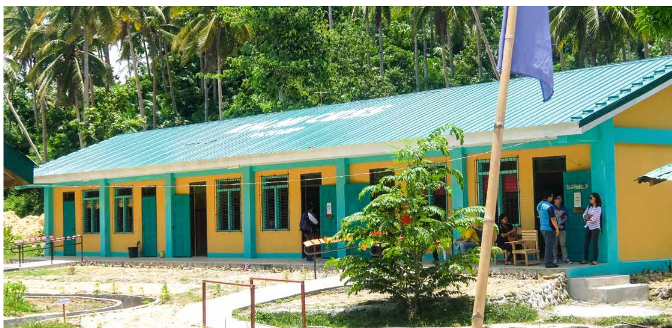
A newly built three-classroom school building/evacuation centre constructed by men and women in Sorsogon Province
