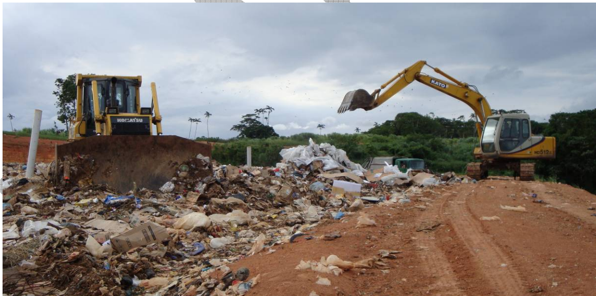
Figure 2: Operations at Bouffa Landfill in Port Vila
