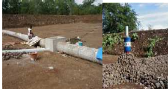
Leachate collection pipe Gas venting pipe
