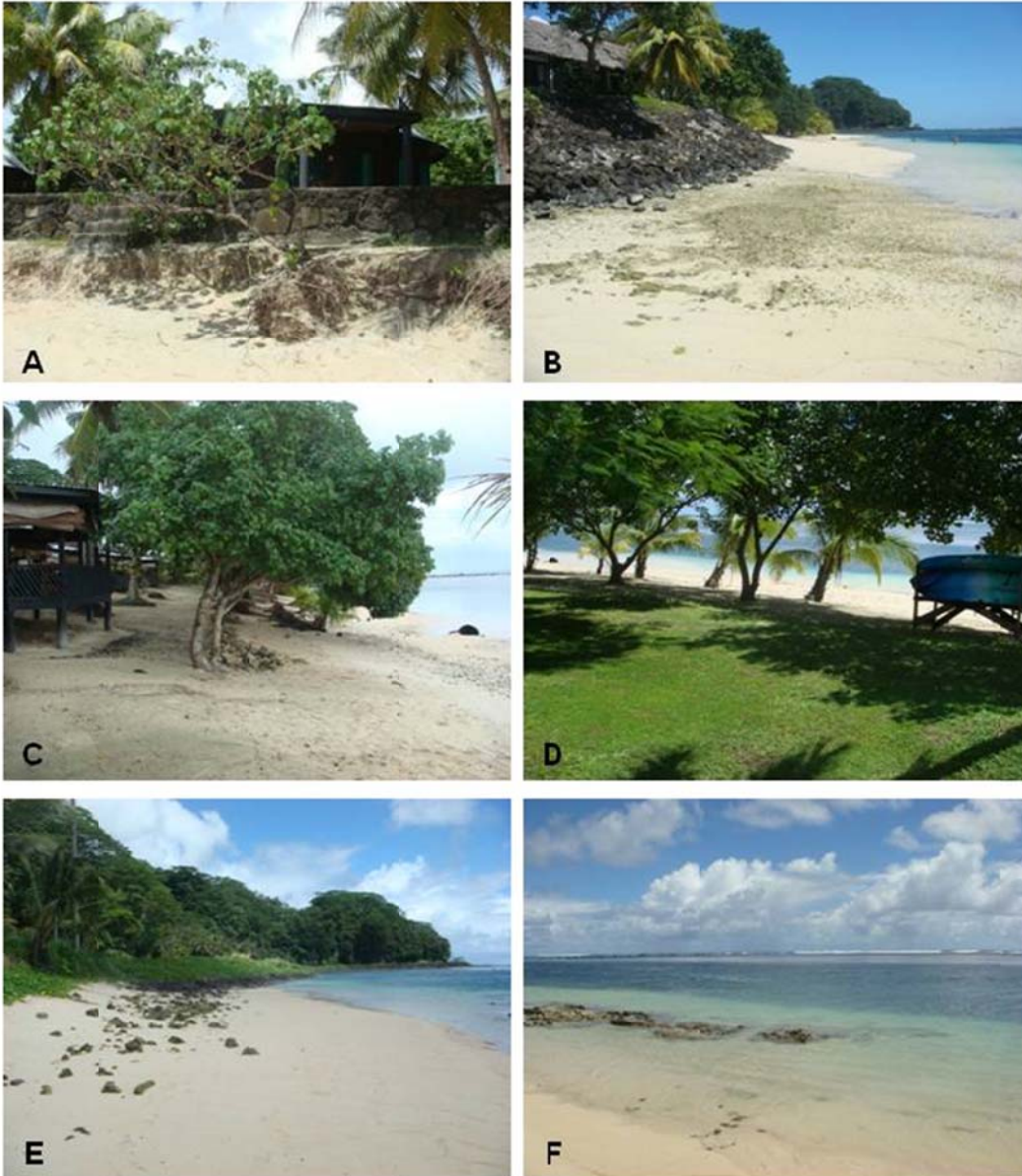
Figure 5. Site features as of April 2013. A) The villas are protected by a retaining wall and tree roots, which stabilize sediment but are being exposed by erosion. Concrete steps allow foot traffic to erode the upper beach. B) The rock revetment protecting new suites is uncemented, allowing large rocks to escape and damage coral. Freshwater flows from beneath the revetment. C) Eurofales are fronted by trees and open beach. D) On the western edge, the beach tapers to meet the seawall protecting the coastal road. The upper beach is covered by fue. E) West of the rock revetment, an open grass-covered lawn slopes gently to the beach, with no erosional scarp along the upper beach. F) Beachrock provides coastal protection, but is removed for aesthetic purposes.
