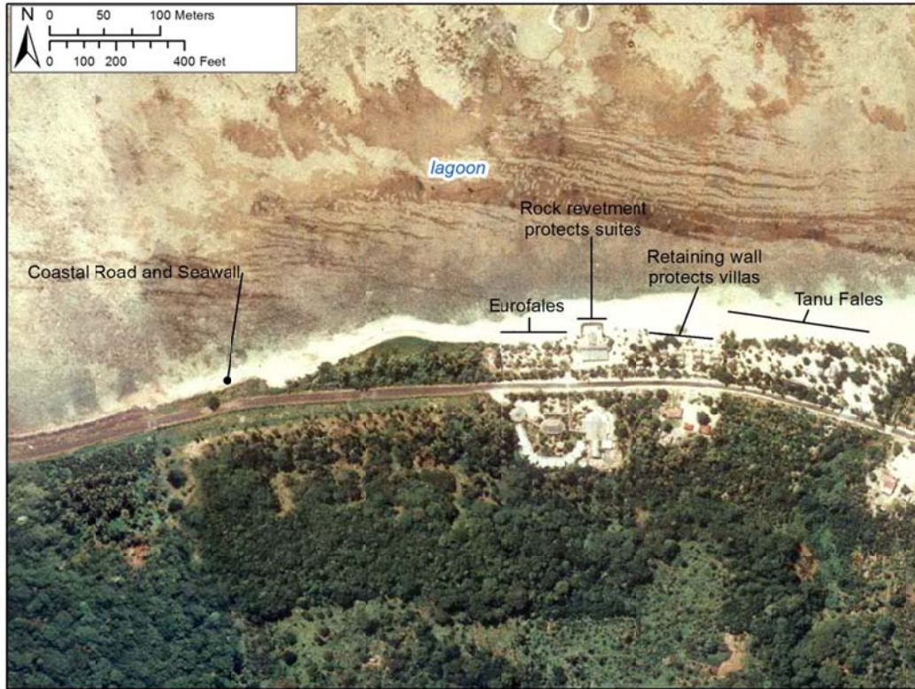
Figure 4. Structures at Stevensons Resort include Eurofales, new suites protected by an uncemented rock revetment, and older villas protected by a retaining wall and tree roots. The site is bounded to the west by a seawall that protects the coastal road, and to the east by another beach accommodation. Photo of ground conditions in 2004 courtesy of SPREP.
