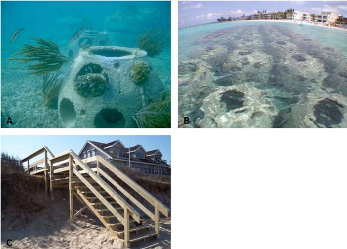
Figure 7. Alternatives considered included nearshore and beach structures including A) underwater reef balls that would provide marine habitat and B) as a group, would reduce incoming wave energy and associated shoreline erosion, and C) stairways that would reduce foot traffic and associated sediment loss on the upper beach. Photos of reef balls from Harris (2009).
