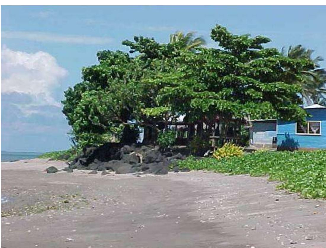
Village seawall in front of church house at Tafitoala showing degree of erosion around the end of the wall.
