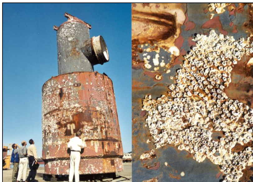
Figure A5-4: Examples of fouling species on floating infrastructure associated with offshore industries (Source: S Raaymakers).
