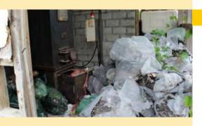
Through PacWaste, inadequate or nonoperational incinerators such as this one at Tungaru Hospital on Tarawa, Kiribati will be replaced with new and efficient equipment to protect the health of people and the environment. Photo: Trevor Thornton
