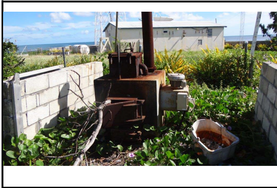
Photo 7: Old ruined incinerator at Niu'ui Hospital, Lifuka Island, Ha'apai Group, Tonga (taken 15/05/2014 by Geoff Latimer ref:DSC04662)
