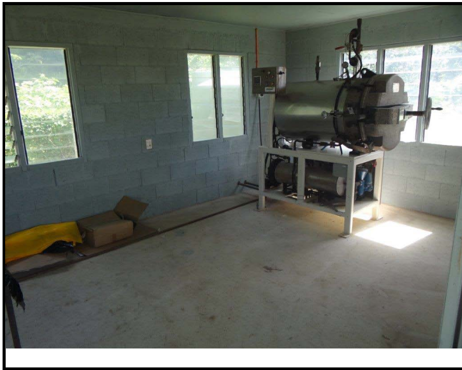
Photo 7: Autoclave (for waste treatment) at Vaiola Hospital, Tongatapu, Tonga (taken 31/03/2014 by Geoff Latimer ref:DSC03867)
