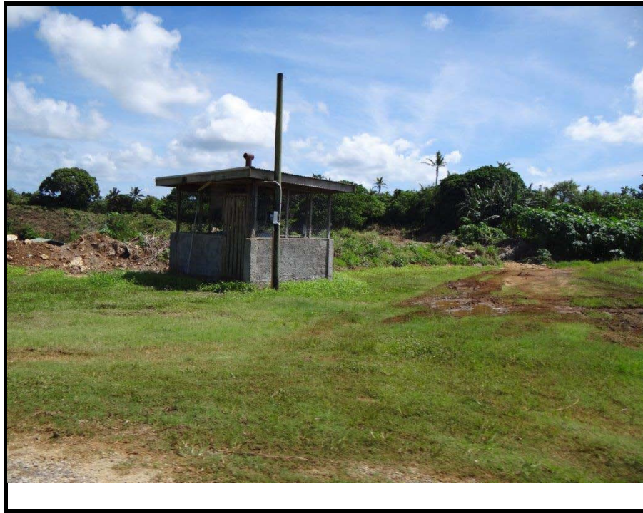
Photo 5: Incinerator at Tapuhia Landfill, Tongatapu, Tonga (taken 31/03/2014 by Geoff Latimer ref:DSC03878)
