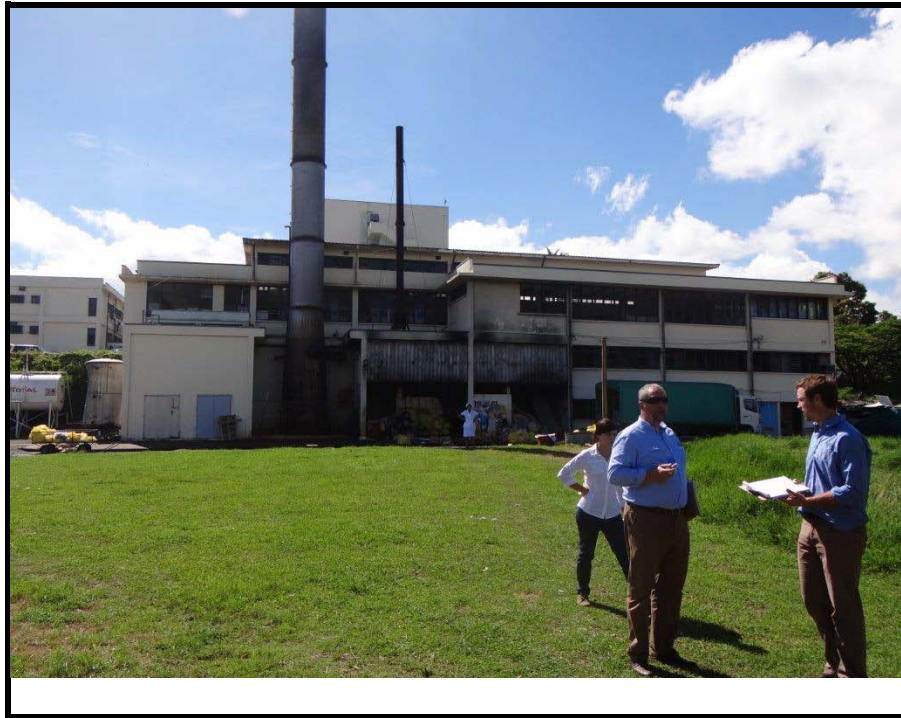
Photo 9: Main incinerator and boiler building, Lautoka Hospital, Fiji (taken 24/3/2014 by Geoff Latimer ref:DSC03600)
