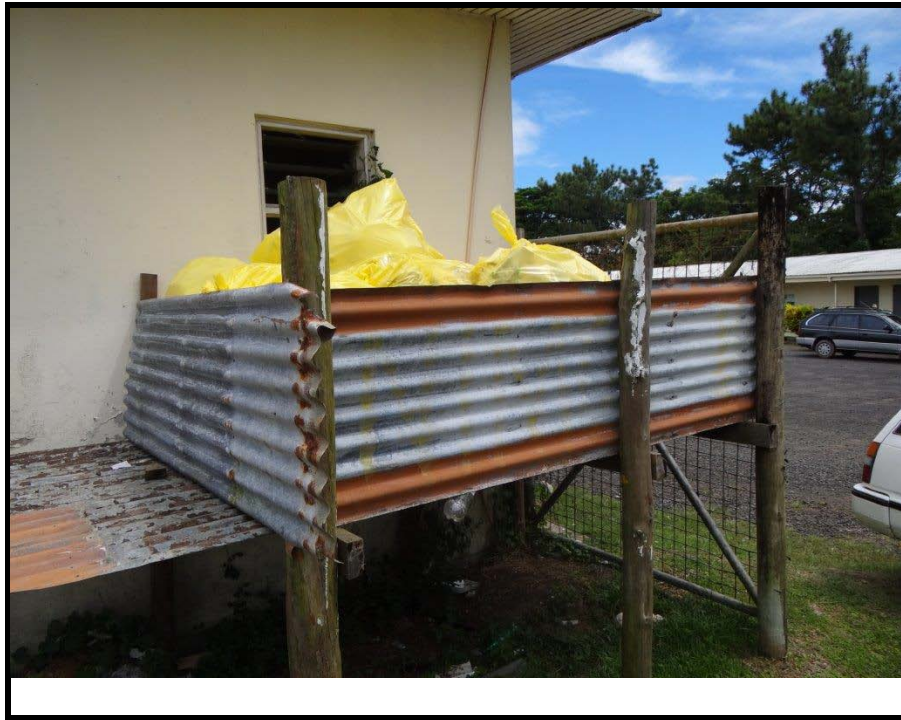
Photo 3: Storage enclosure for healthcare waste bags prior to collection for incineration, Sigatoka Hospital, Fiji (taken 25/03/2014 by Geoff Latimer ref:DSC03659)
