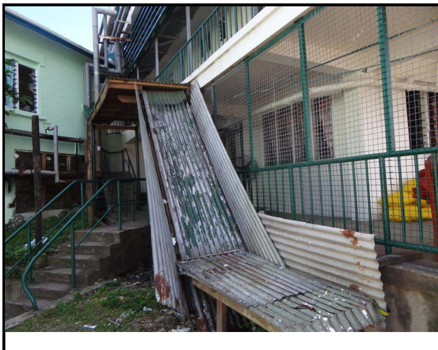
Photo 6: Slide structure for transfer of healthcare waste bags, CWMH Suva, Fiji (taken 26/3/2014 by Geoff Latimer ref:DSC03694)
