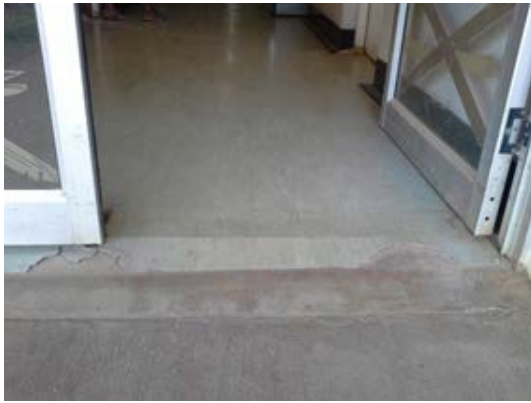
Photo 7 – Port Vila Central Hospital
