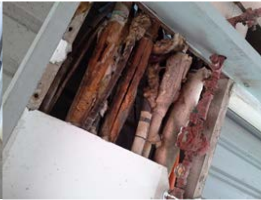
Photo 8 – Port Vila Central Hospital
