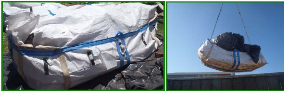
Photos 17 and 18: Asbags in Use
