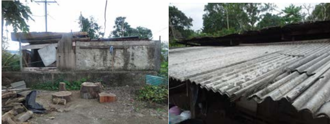
Photos 13 and 14 – Residence in Luganville
