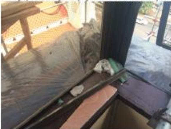
Photograph 2: Damaged roofing material observed on 6 th floor of John Williams Building.
