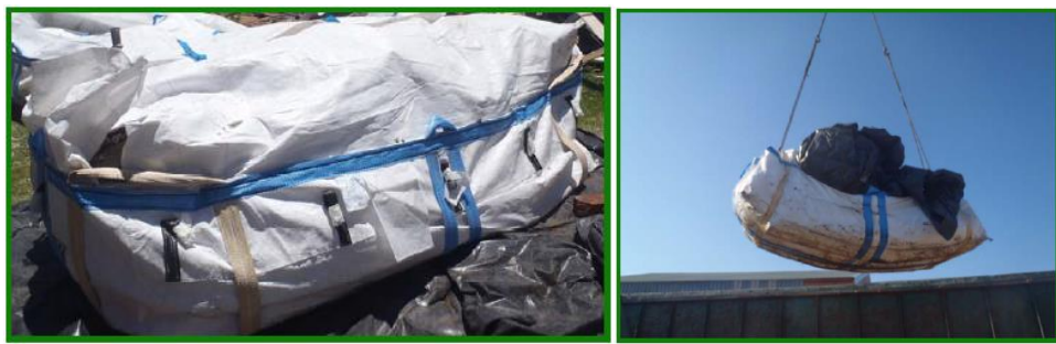
Photos 11 & 12: Asbags in use
