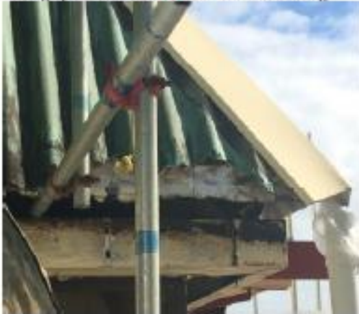
Photograph 2: Damaged roofing material observed on 6 th floor of John Williams Building.
