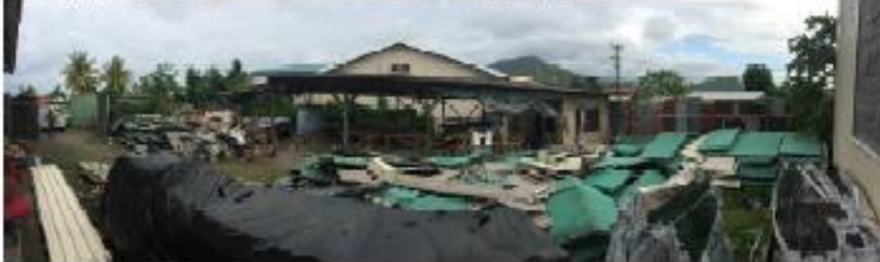
Photograph 5: View south west to south east in SPC compound;
