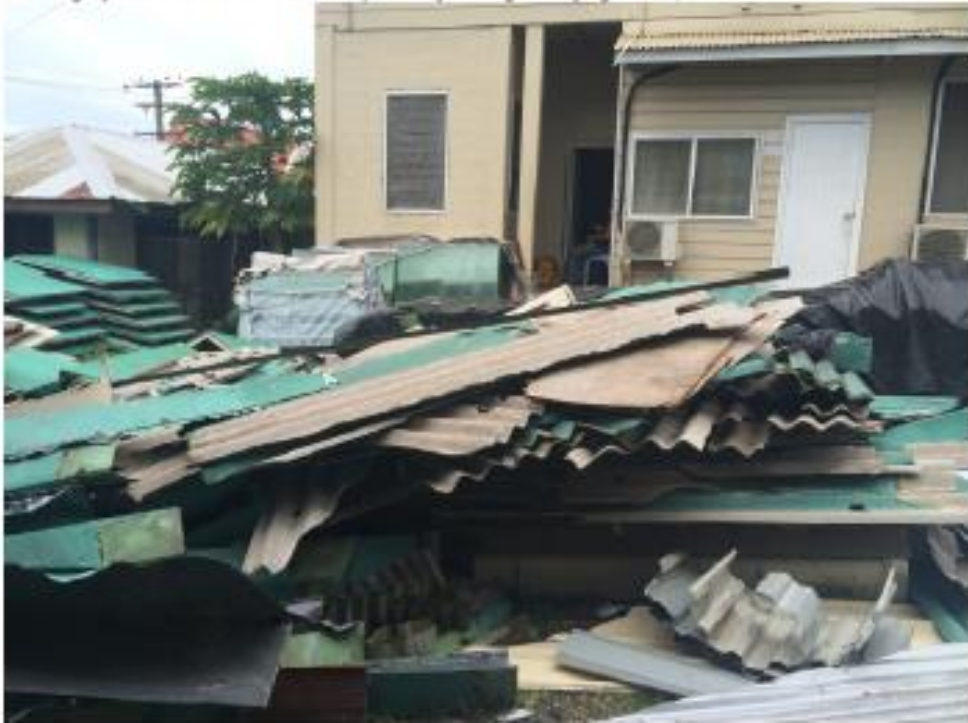
Photograph 6: View north in SPC compound of damaged roofing sheets;
