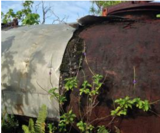
Photo 27: Close-up of Tank A Lagging
