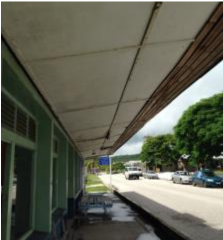
Photo 15: Alofi Bread Shop Soffits
