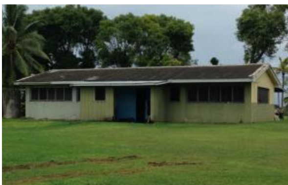
Photo 9: Honey Processing Building Roof
