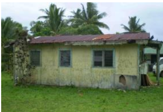
Photos 5-6: Houses with Asbestos Cladding
