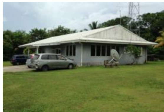
Photo 10: Niue Broadcasting Cladding/Soffits
