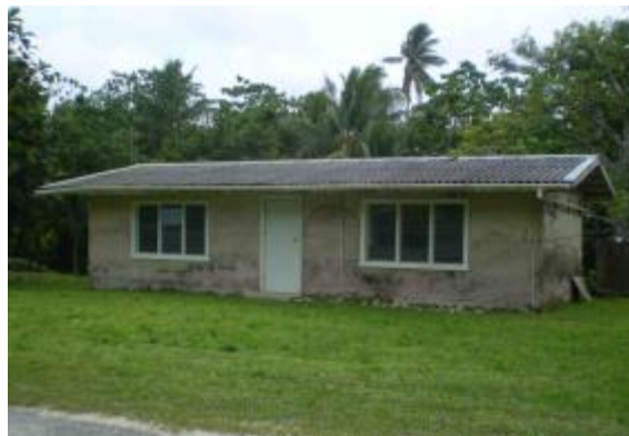
Photos 1-4: Houses with Asbestos Roofs
