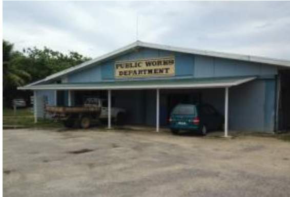
Photo 7: Public Works Department – Cladding Front and Sides
