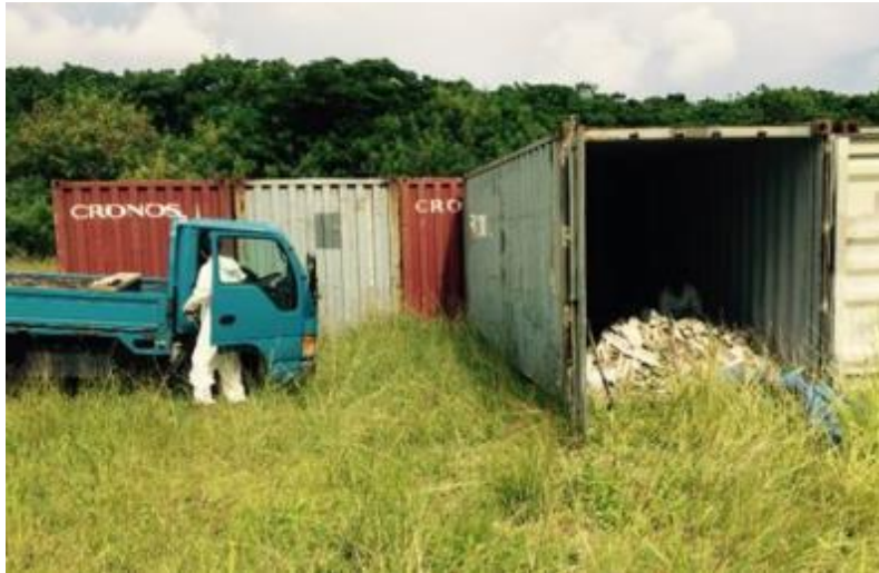
Photo 32: Asbestos Processing Operations
