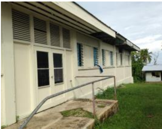
Photo 19: Alofi South Hall Cladding
