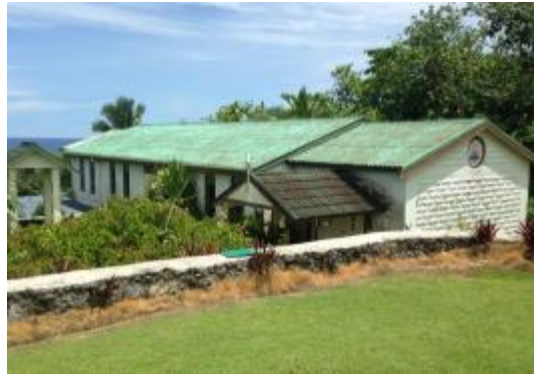
Photo 24: Catholic Church Roof
