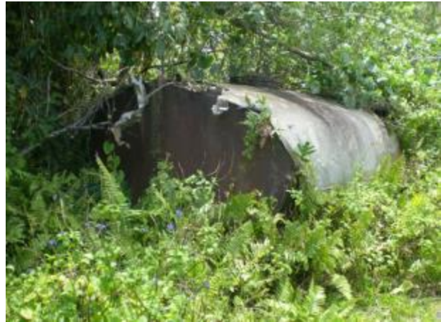
Photo 28: Bitumen Tank at Hui Hui
