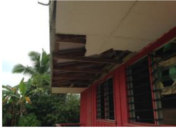
Photos 11-12: Primary School – Cladding and Soffits
