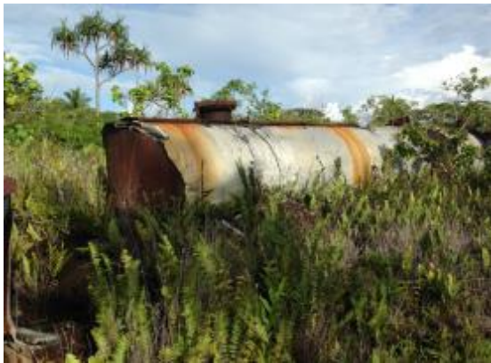
Photo 25: Reservoir Bitumen Tank A
