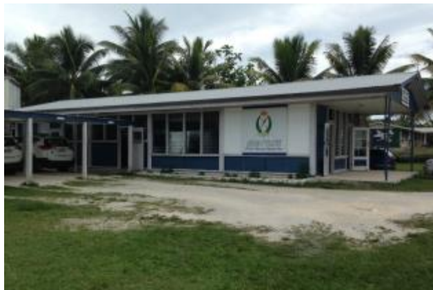
Photo 16: Police Station Cladding
