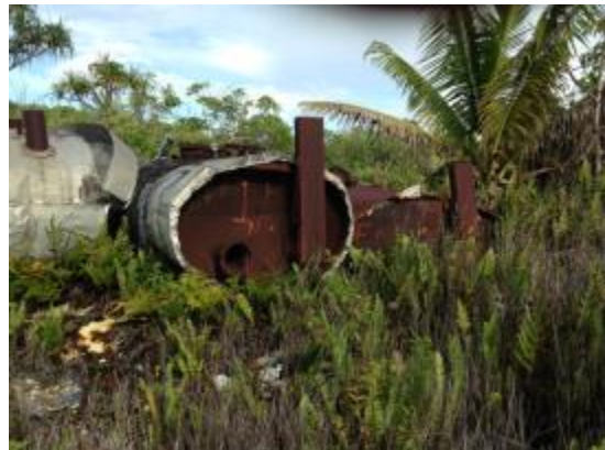
Photo 26: Three Reservoir Bitumen Tanks
