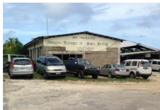
Photo 22: St Joseph's/Peta Paints Roof and Cladding
