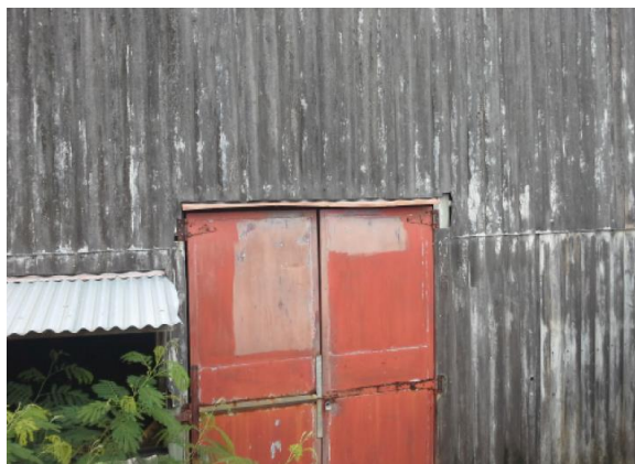
Photo 14 – Fishing Corp Generator Bldg
