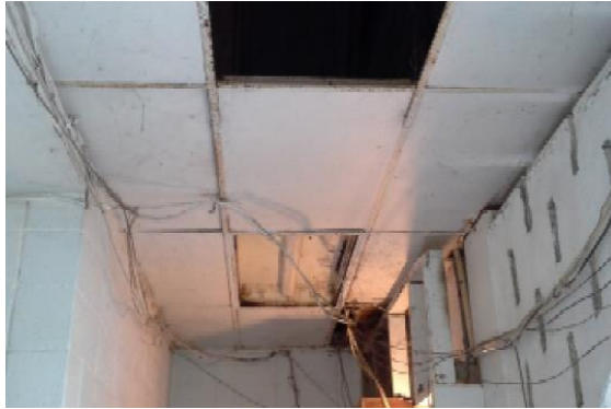
Photo 10 – State Court Ceiling
