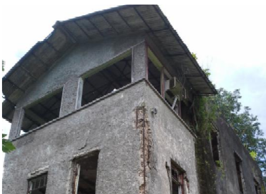
Photo 13 – Botannic Garden Spanish Bldg
