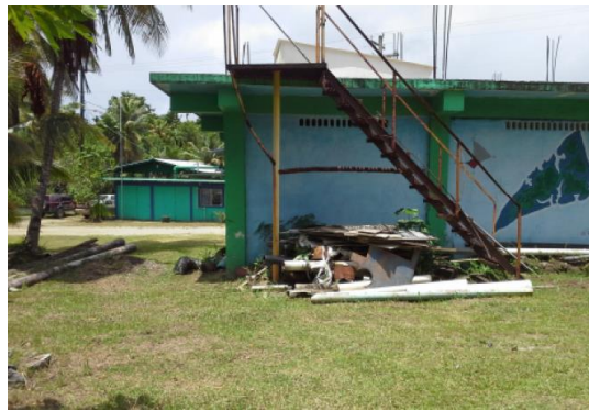
Photo 6 – Yap Water Treatment Plant
