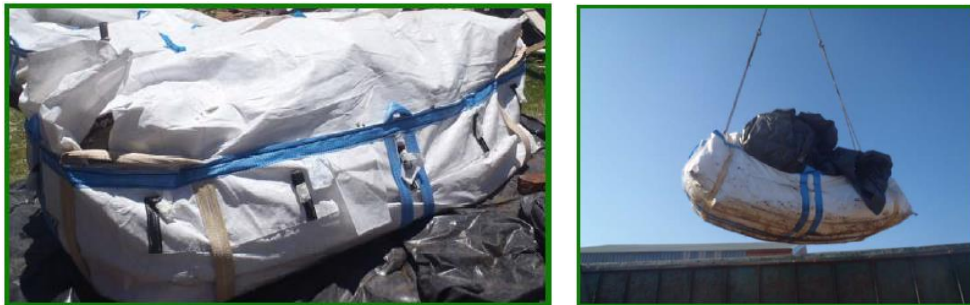
Photos 21 & 22: Asbags in use
