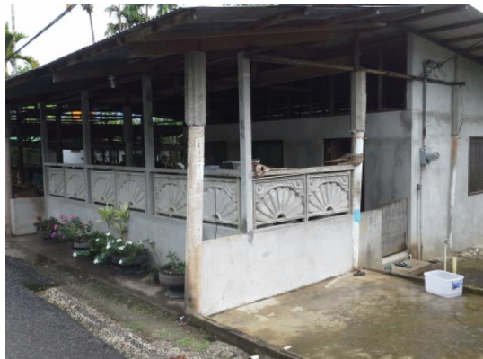
Photo 18 – Residence – AC Pipe Columns
