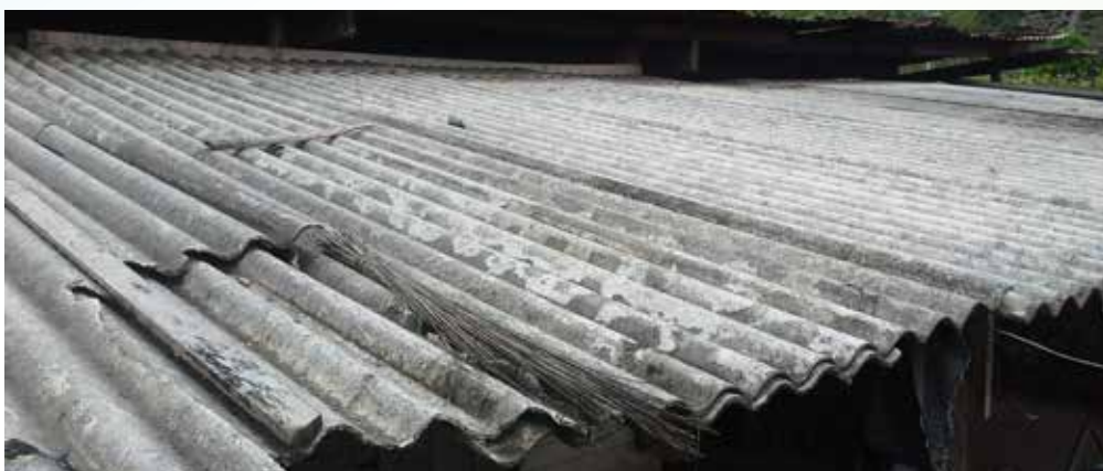
Corrugated asbestos cement roofing, pictured here on a building in Vanuatu, is relatively easy to recognise through visual inspection. Photo: PacWaste
